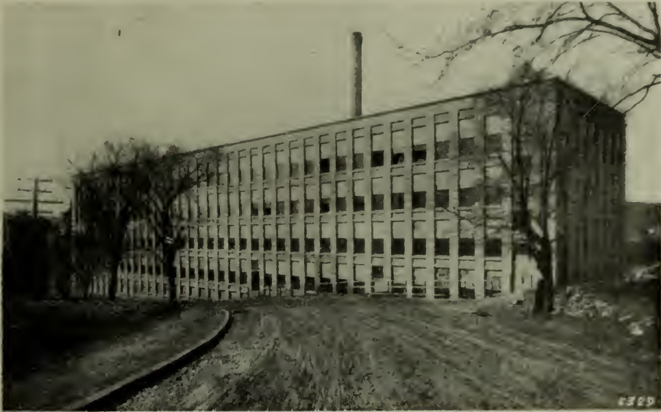
FIG. 4. A MILL BUILDING.
